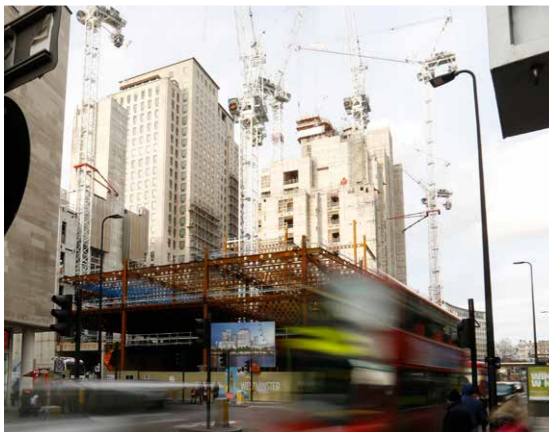
Southbank Place in construction. Photo credit: Jason Ellis
